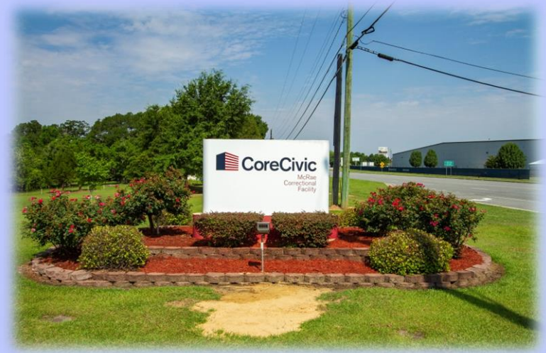
Core Civic-McRae Correctional Facility
