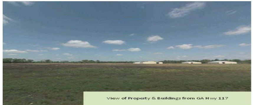
View of Buildings from GA Hwy 117
