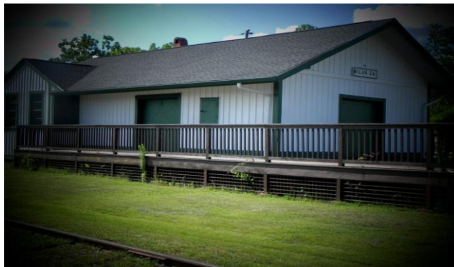
Historic Train Depot
